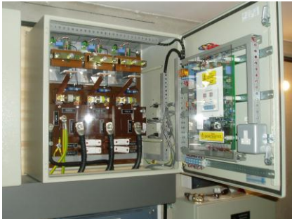
Above is a Z-LYNK HPT Controller measuring just 600*600*400 (H*W*D mm)
